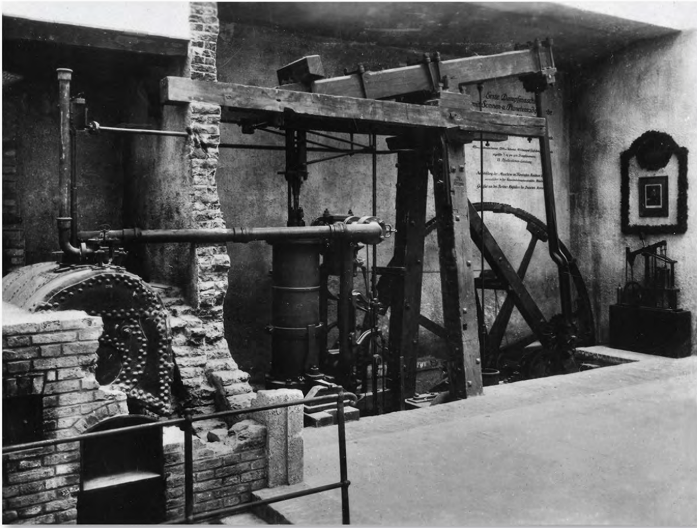
Figure 11-1: Watt's engine was effective at transforming heat energy into mechanical power.
